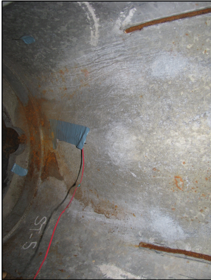
(a) Dent viewed from inside the pole with additional steel ribs on either side of dent
