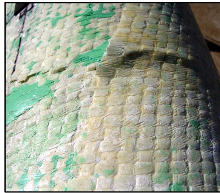
(b) FRP buckling failure
