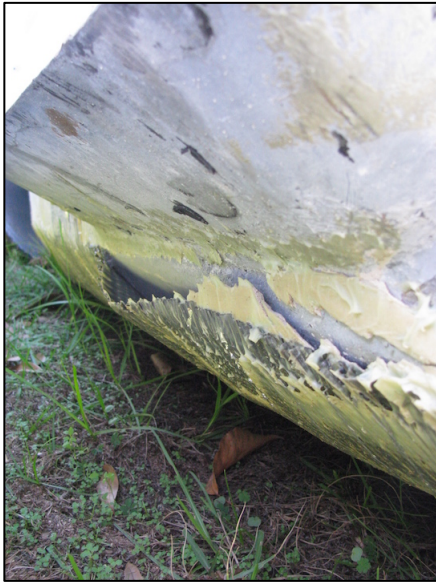
(a) Delamination and separation of the transverse wrap near the access port
