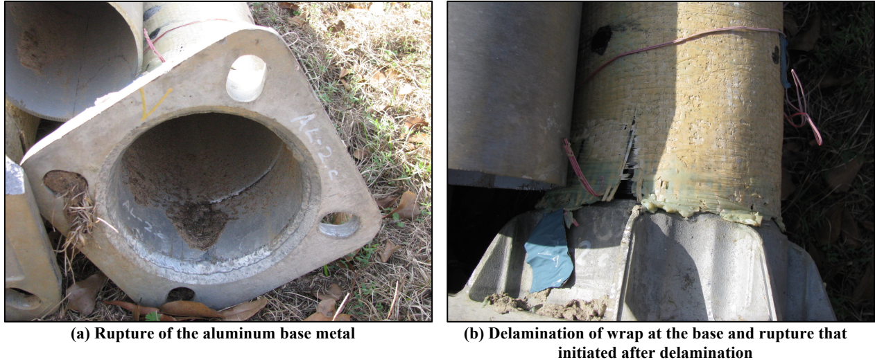
Figure 197. AL-2.c after testing
