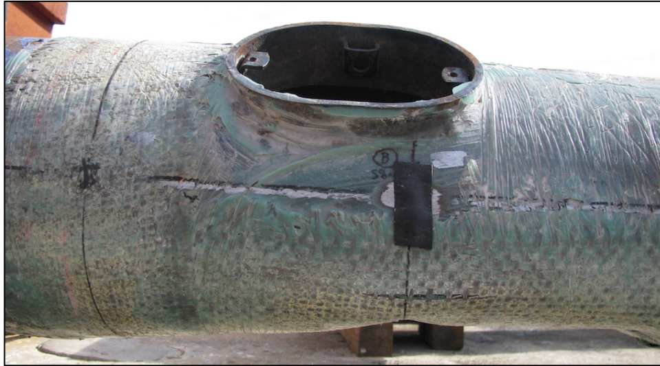
(a) Deformation of the access port and rupture in FRP
