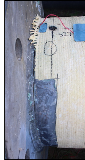
(b) Crack propagated nearly full depth
