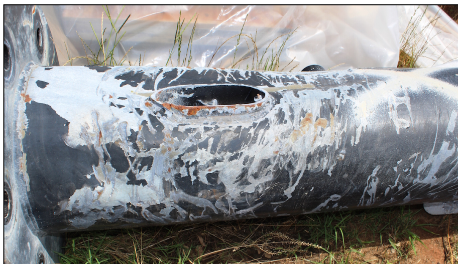
Figure 135. Original vehicular damage to access port region in FD-1
