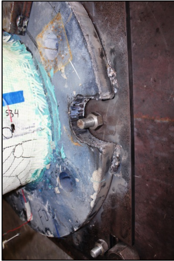
(a) Ruptured pole base plate welds near bolt on west side of pole
