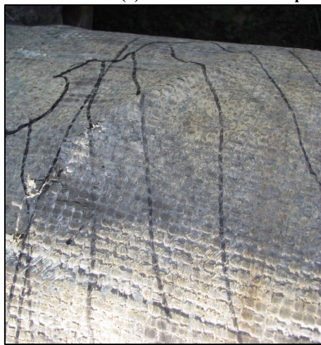
(b) Compression wrap failure
