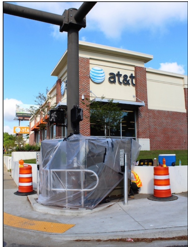
(b) Protective plastic tent during installation
