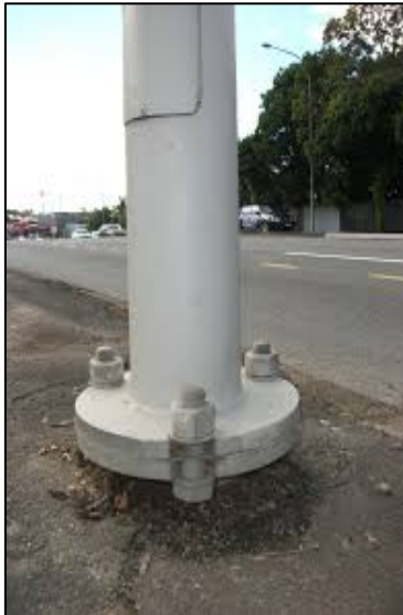
Figure 204. Typical light pole base
