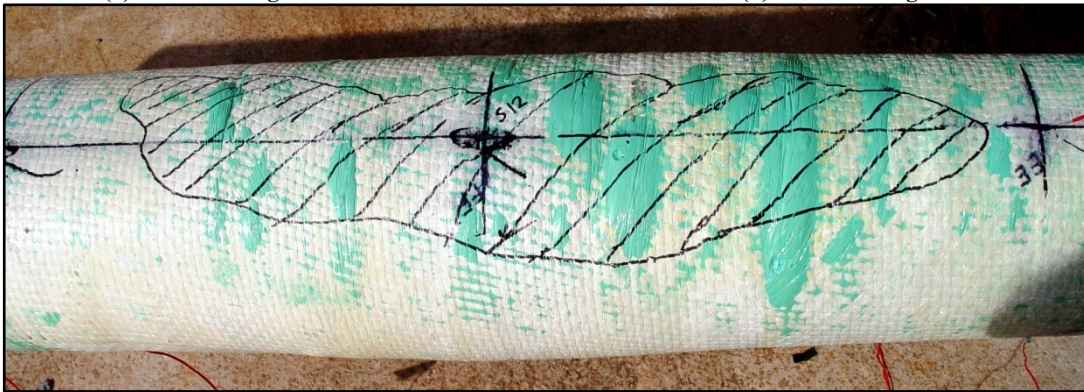
(c) FRP debonding from tension face
