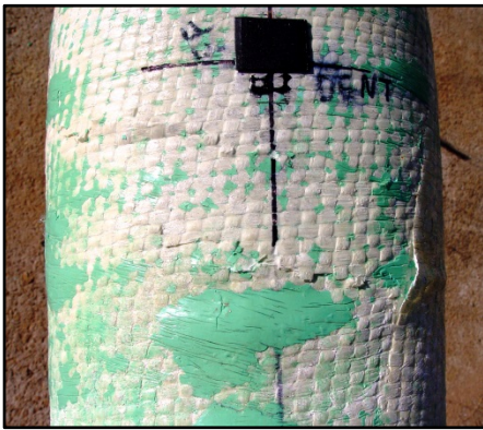
(a) FRP buckling failure
