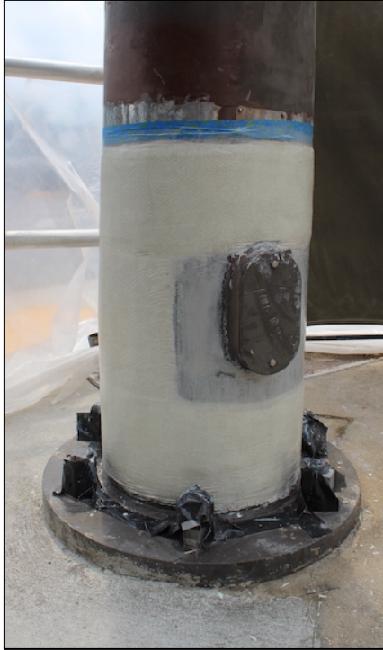
(a) Wrapped pole before painting
