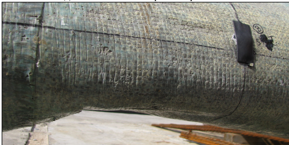
(b) Local deformation and rupture of FRP in impact head region Figure 248. IM-1 post-test state of repair material at impact location
