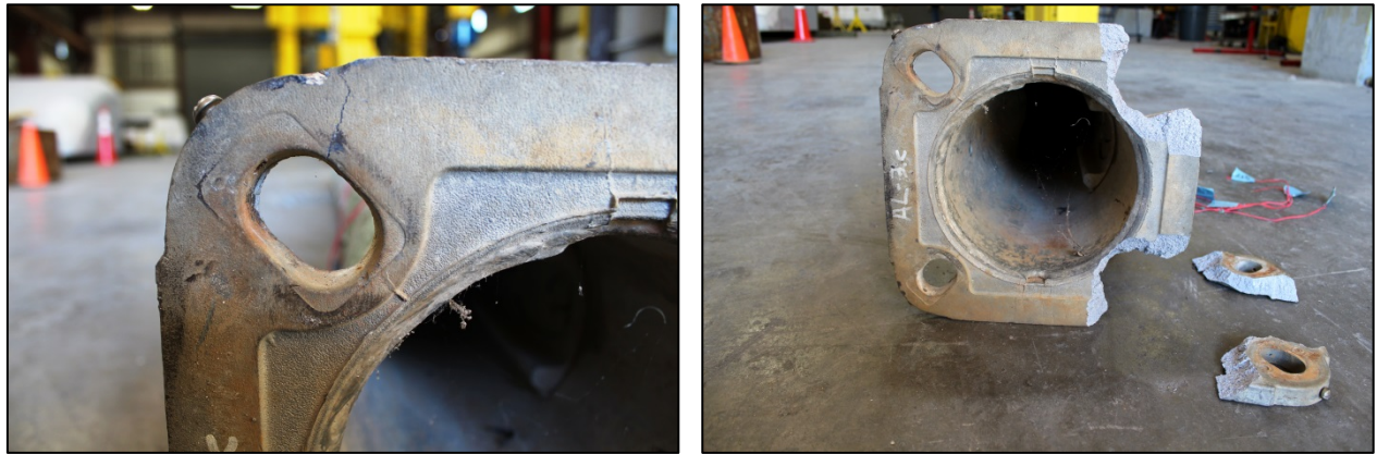
(a) Fractured base plate
