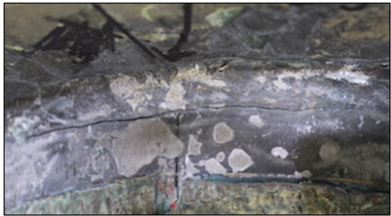
(b) Crack detail
