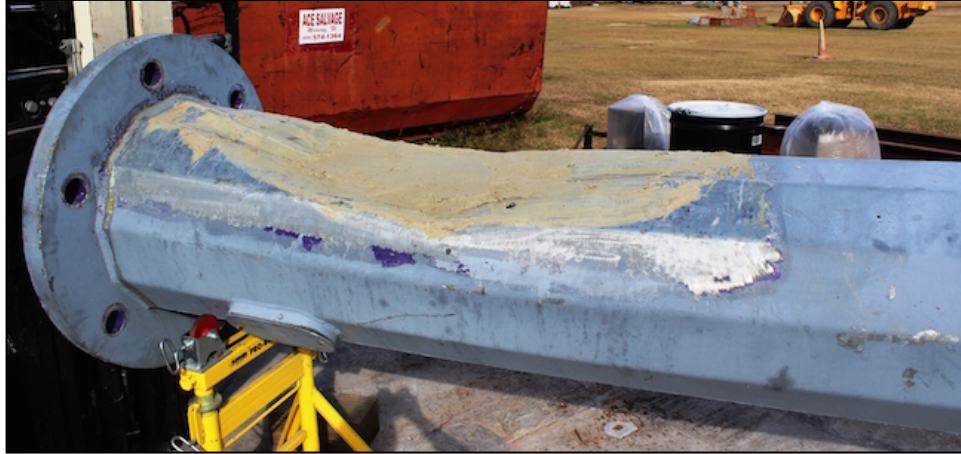
Figure 249. IM-2 dent cavity volume requiring fill material
