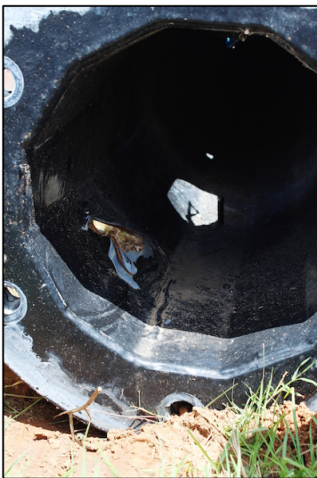
(a) Interior view showing puncture
