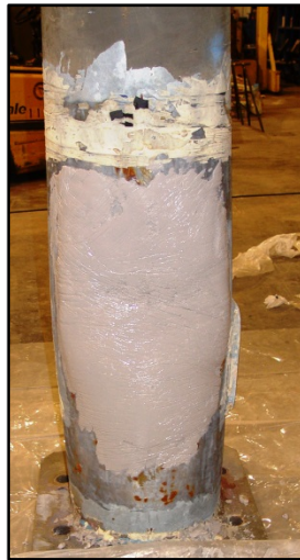
Figure 12. Sikadur 31 dent fill 1
