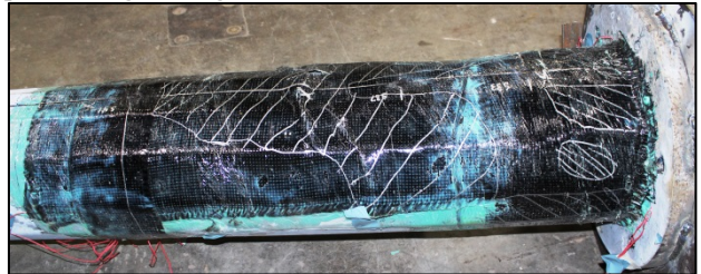
(c) East face – debonded and ruptured FRP
