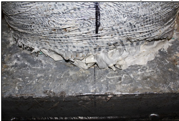
(b) FRP potentially debonded near the base and accumulation of resin near base flange
