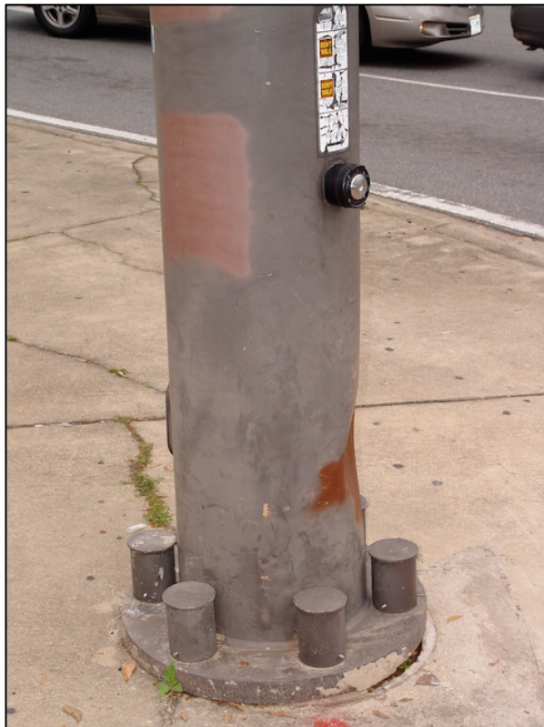
(a) Pole damage at base
