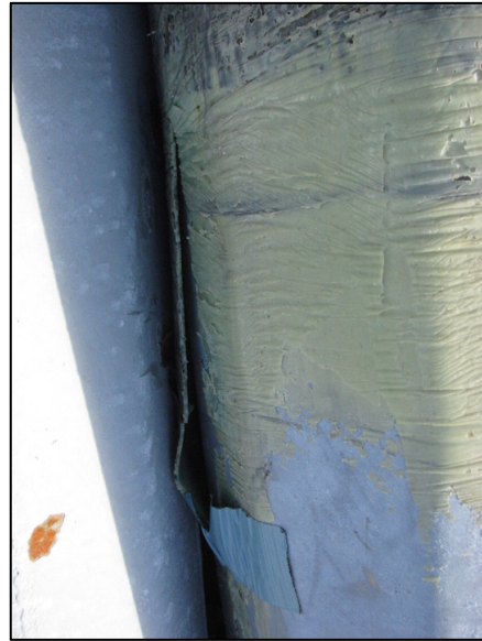
(b) Delamination and separation of the transverse wrap on the face opposite to the access port
