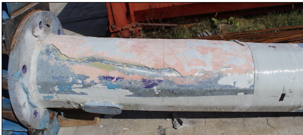
(a) Fill material after impact with wrap removed
