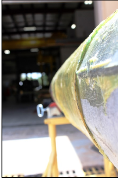
Figure 104. Voids between composite wrap and steel substrate
