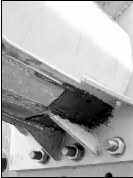
Figure 5. CFRP reinforcement on steel monopole (Schnerch & Rizkalla, 2004)
