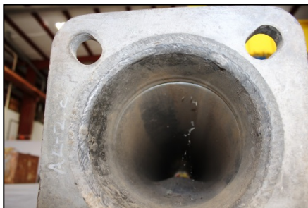
(b) Failed base plate connection
