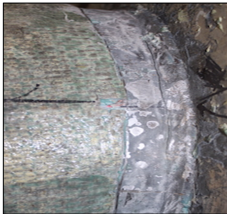
(a) Cracking at weld toe
