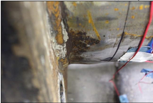
(b) Buckled steel 2 in above base plate
