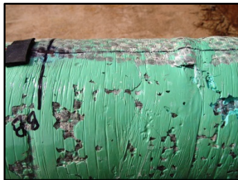
(a) Fiber buckling
