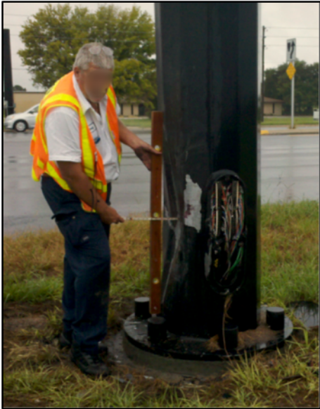
Figure 1. Impact-damaged utility pole
