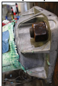
(c) Ruptured fibers and failed base plate connection
