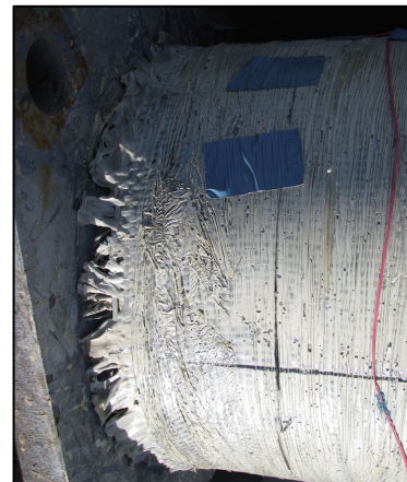
(c) Dilation of the base section and possible debonding
