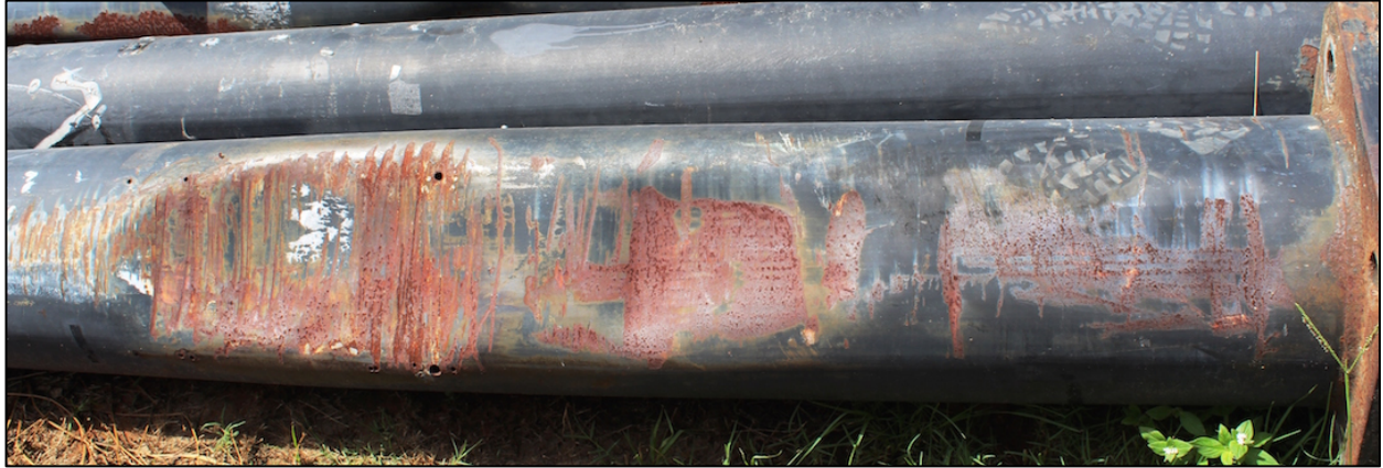
Figure 149. Vehicular dents present in FD-3 prior to repair
