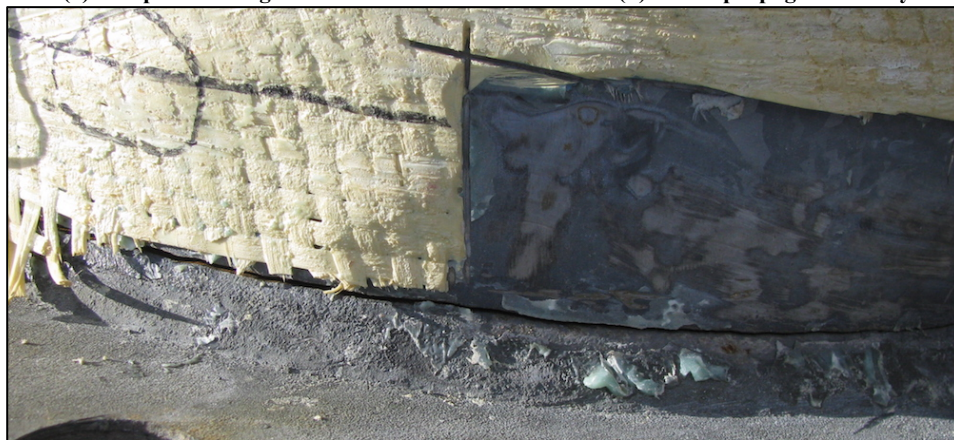
(c) Crack detail
