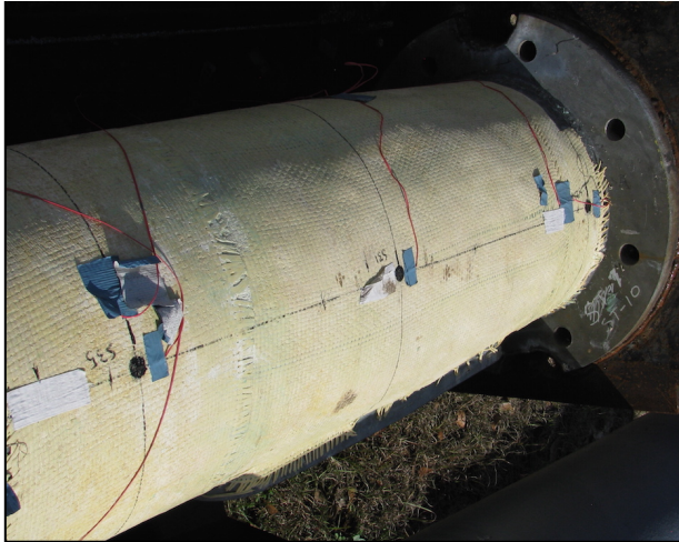
(a) Wrap not damaged
