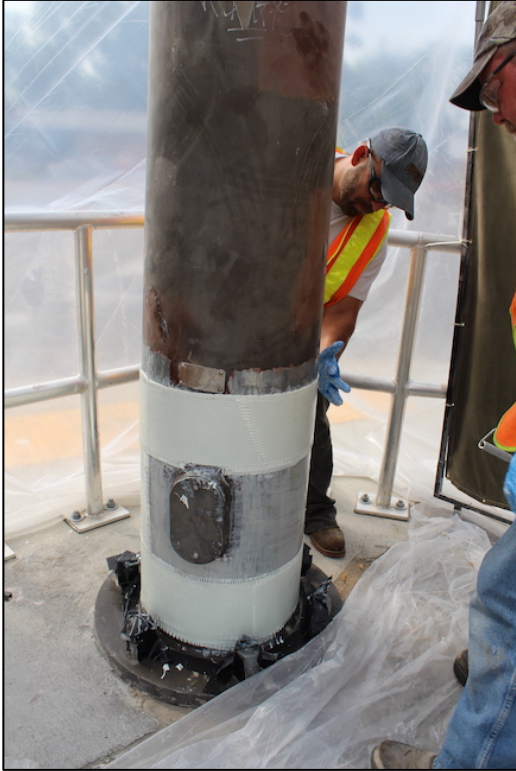
(a) Rolling transverse layer of GFRP
