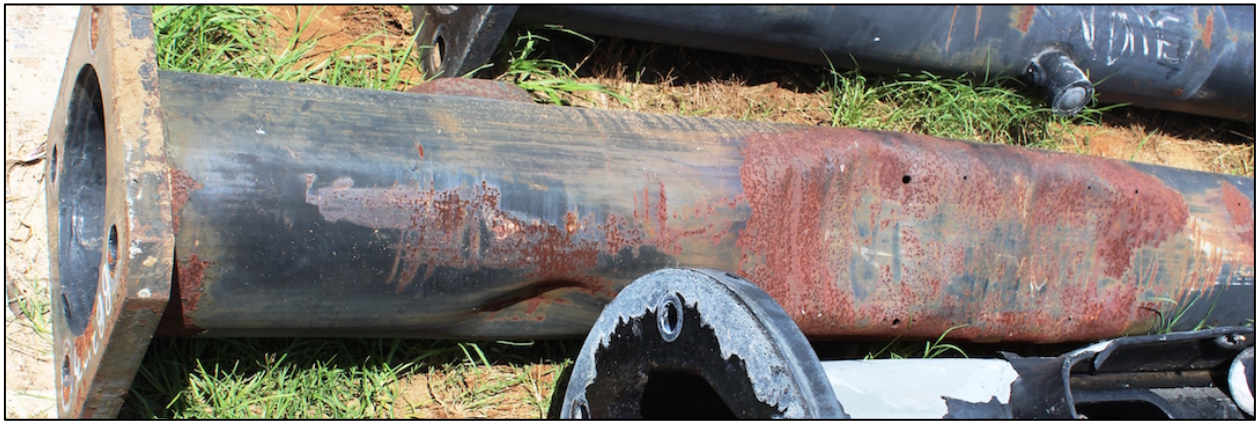
Figure 157. Vehicular damage to FD-5 prior to repair
