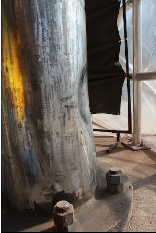
(a) After surface preparation in the repair region
