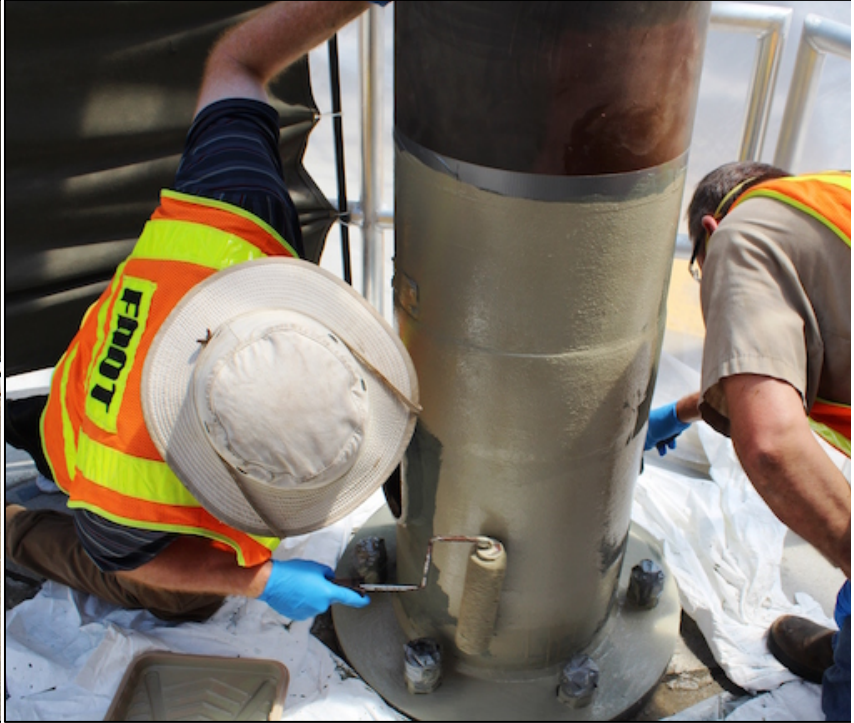
(b) Painting in progress
